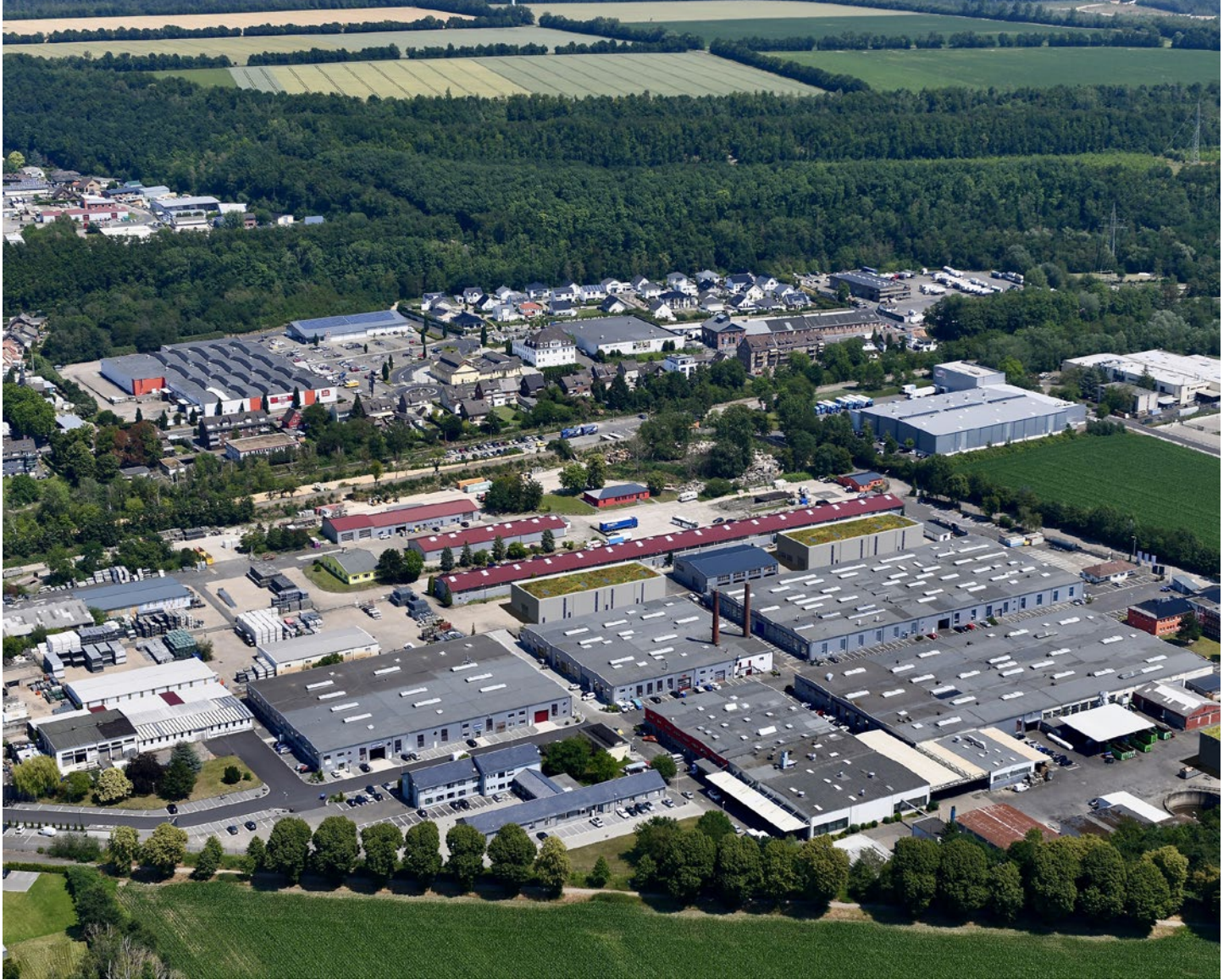
Luftbild des Technologieparks in Bergheim Aerial view of the technology park in Bergheim
